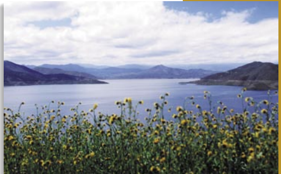
Diamond Valley Reservoir, Metropolitan Water District of Southern California.
