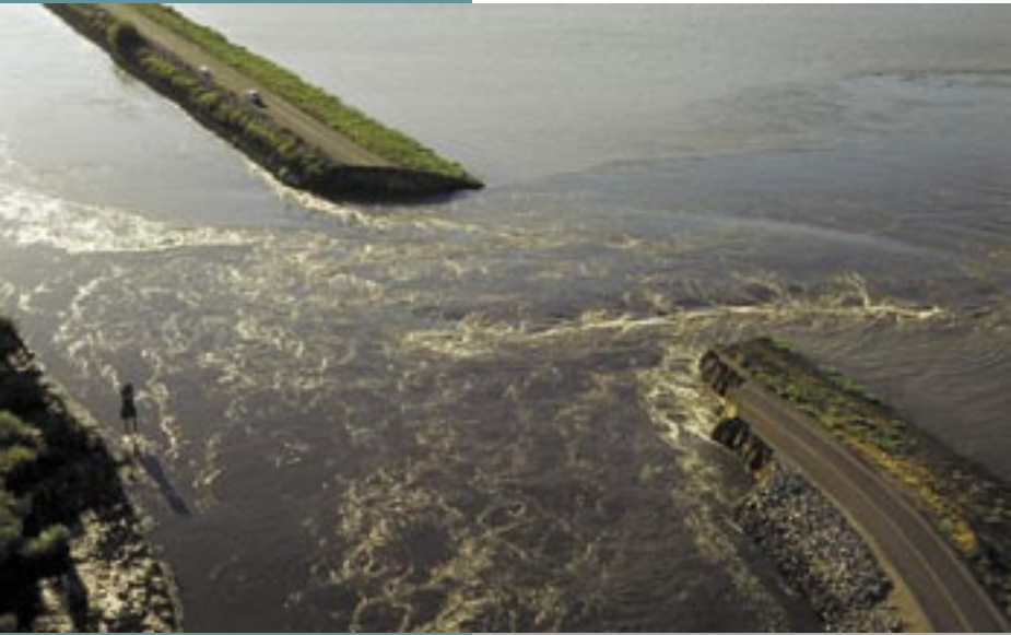
Flooding after Jones Tract levee break in June 2004.
