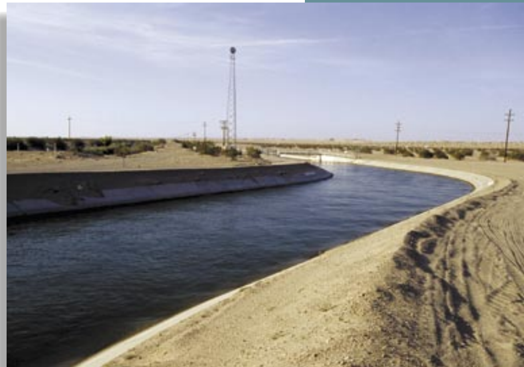
Colorado River Aqueduct Canal.
