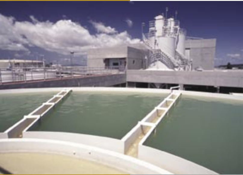
North Richmond Water Reclamation Plant, East Bay Municipal Utility District.
