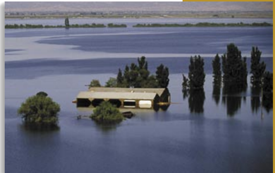
Flooded structure resulting from the Jones Tract levee break, June 2004.
