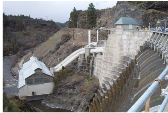
Figure 2-6. Powerhouse at Copco No. 1 Dam
