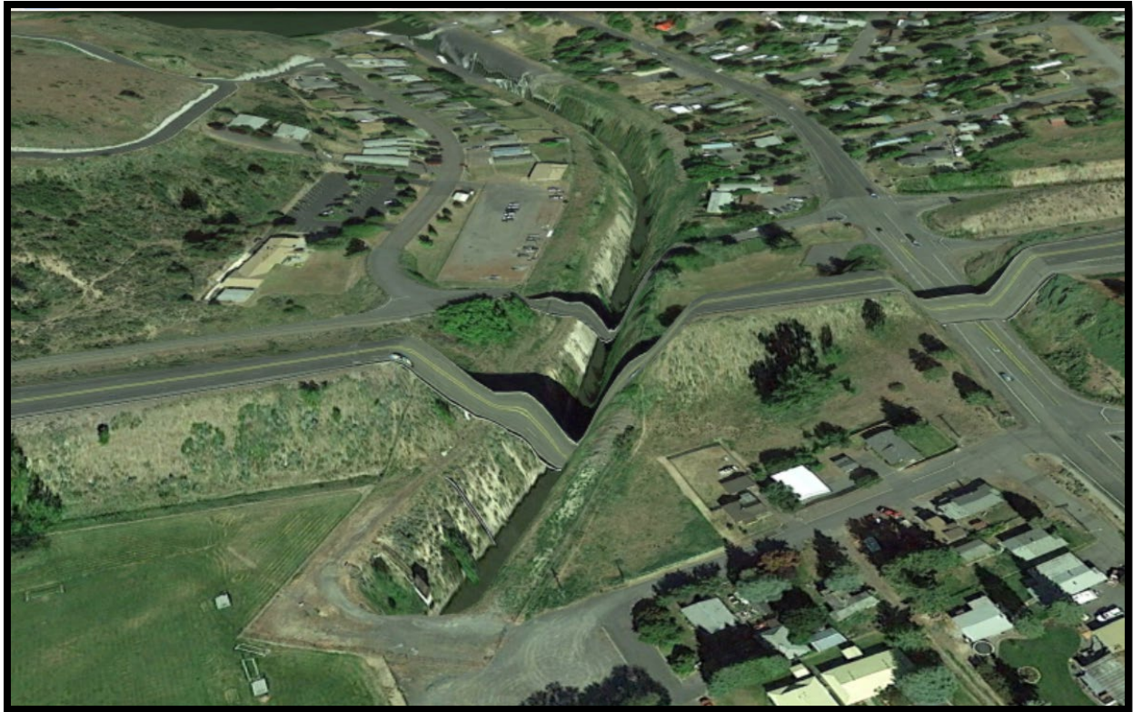
Figure 19 Google Earth Imagery of A Canal from Headworks to Tunnel Entrance
