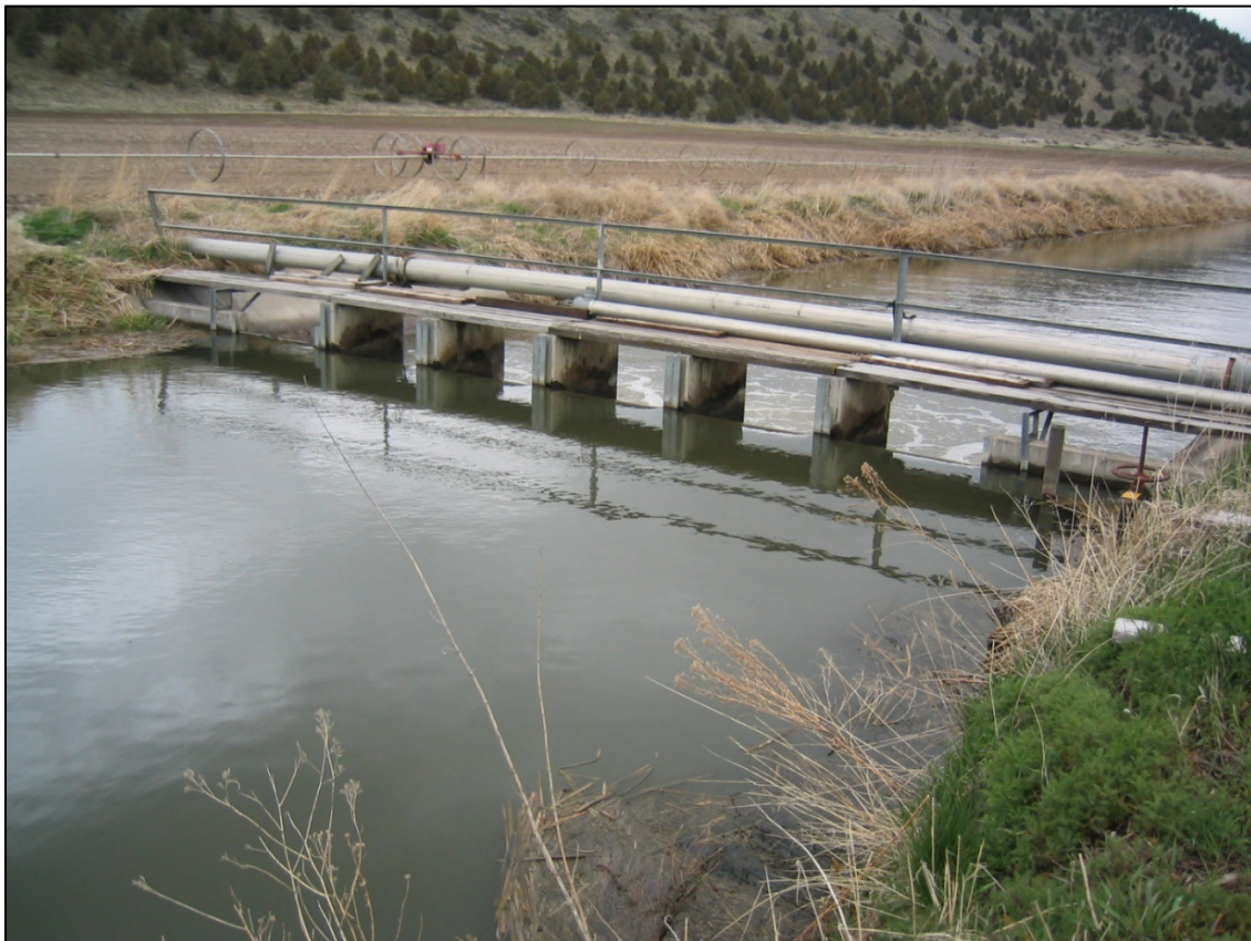
Figure 68 D Canal Weir at Covington Station
