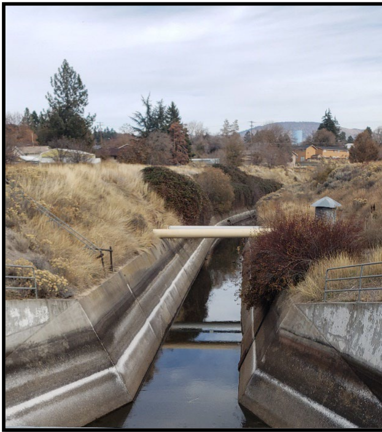
Figure 18 A Canal (looking east) at its Headworks
