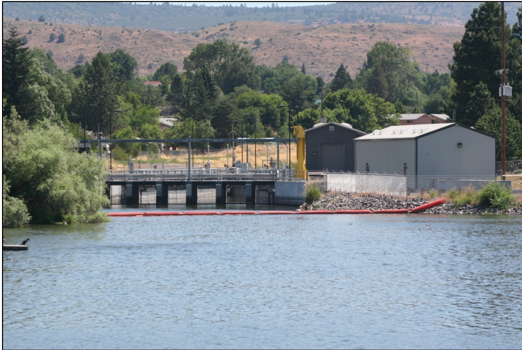
Figure 60 A Canal Headworks
