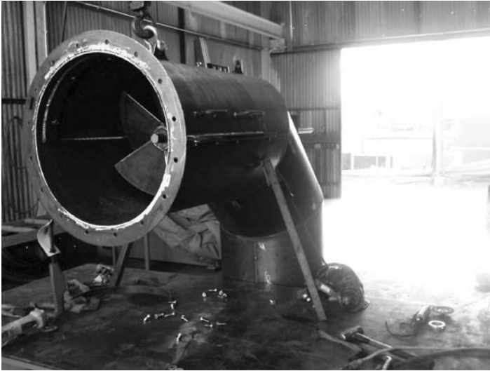
Low-head hydropower turbine for EBID under construction. Photo courtesy of EBID.
