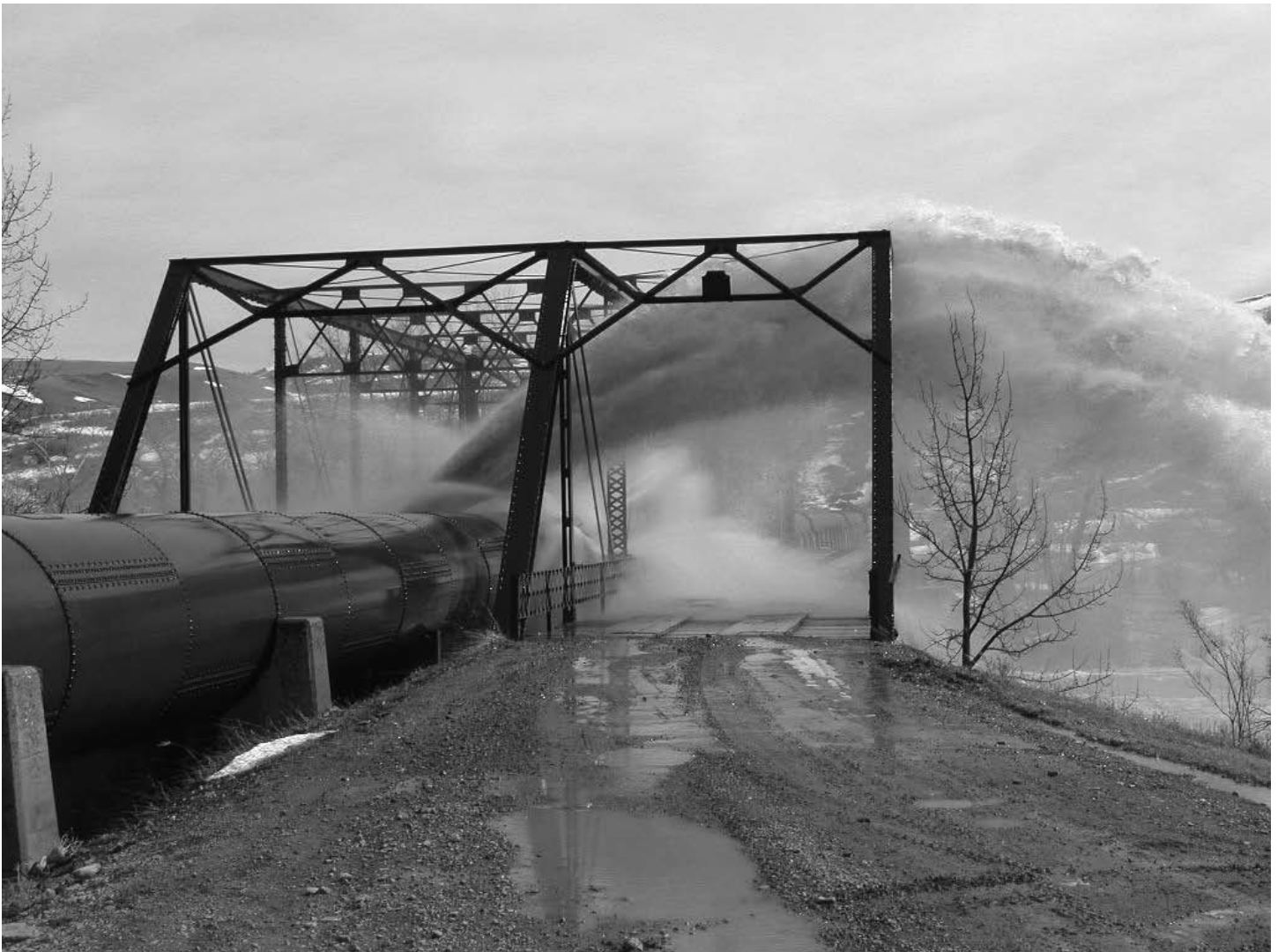
Catastrophic blow-out of one of the siphons along the St. Mary river, resulting in closure of the system for two months, photo courtesy of Larry Mires, St. Mary Rehabilitation Working Group.
