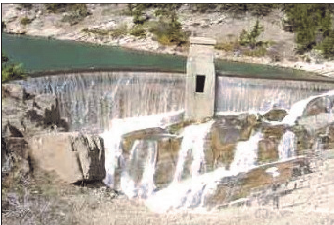
Greenfields Irrigation District's Sun River Diversion Dam in Montana.
