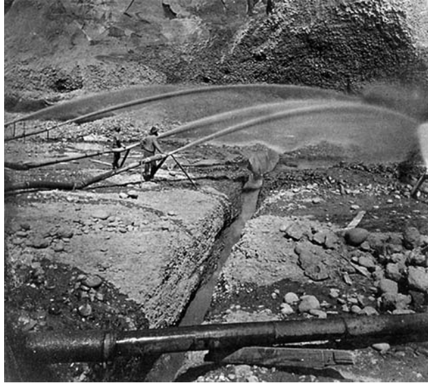
Figure 1.3. Hydraulic mining with high-pressure water hoses in the foothills of the Sierra Nevada. This method of placer mining was invented in California. (Photo by: California Department of Water Resources)
