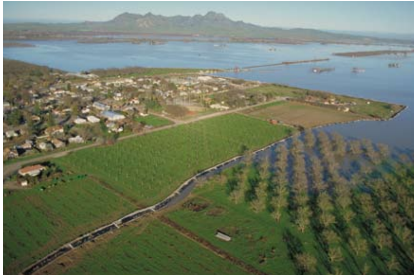
Figure I.2. Levee failures can result in extensive damage to homes and agricultural fields. Flooding also imperils our water supply. (Photo by: California Department of Water Resources)
