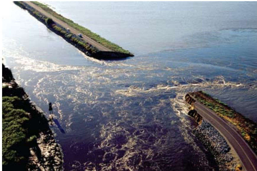
Figure 1.6. The Jones Tract levee failure and flooding of June 3, 2004. The levee was repaired and the Jones Tract restored at an estimated cost of $90 million. (Photo by: California Department of Water Resources)
